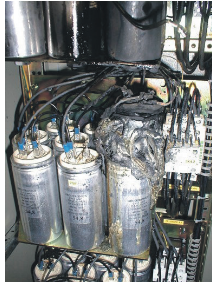
Fig.: Capacitors destroyed due to harmonics
